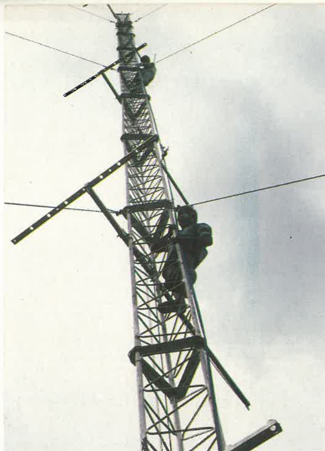
High resolution meteorological instruments installed on a 30-m tower at the I.I.T., Kharagpur, as a part of MONTBLEX-90 programme.
